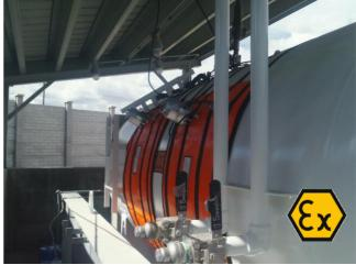
Outdoor Installation example in North America with C1Z1 heating jackets and controllers
